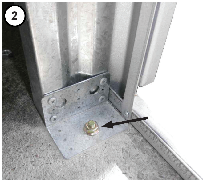
Door stud (Not portal frame) have a single anchor through a BKT17. Fixed by four tek screws.
